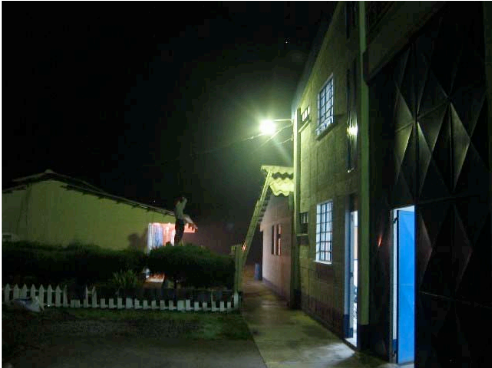
This is me running CAT5 cable to the classrooms...
